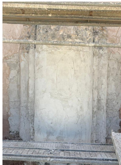
Légende: Completed strengthening system with SikaWrap® FX-50 C
