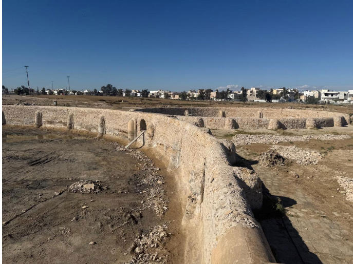
Removal of the original lime-based render.
