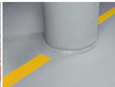
Joints de sol et parking
