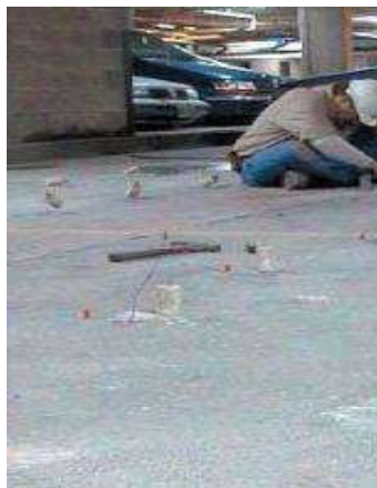
Anodes discrètes instal parking.
