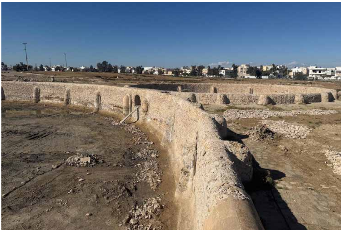
Removal of the original lime-based render.
