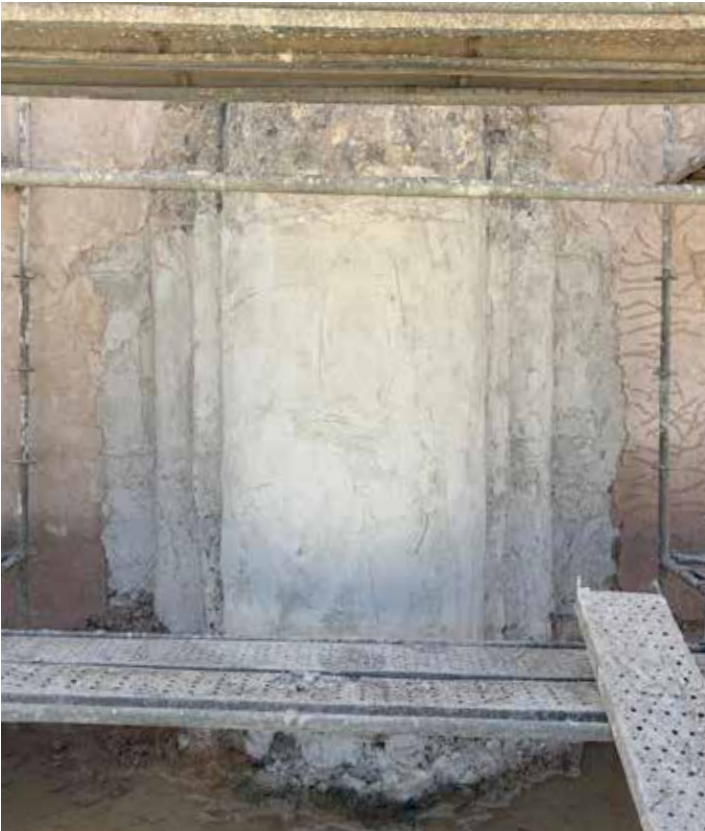
Completed strengthening system with SikaWrap® FX-50 C.
