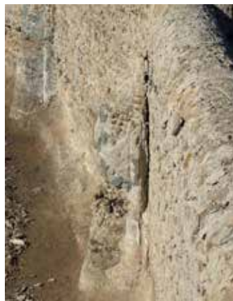
Condition of buttresses showing diagonal cracks.
