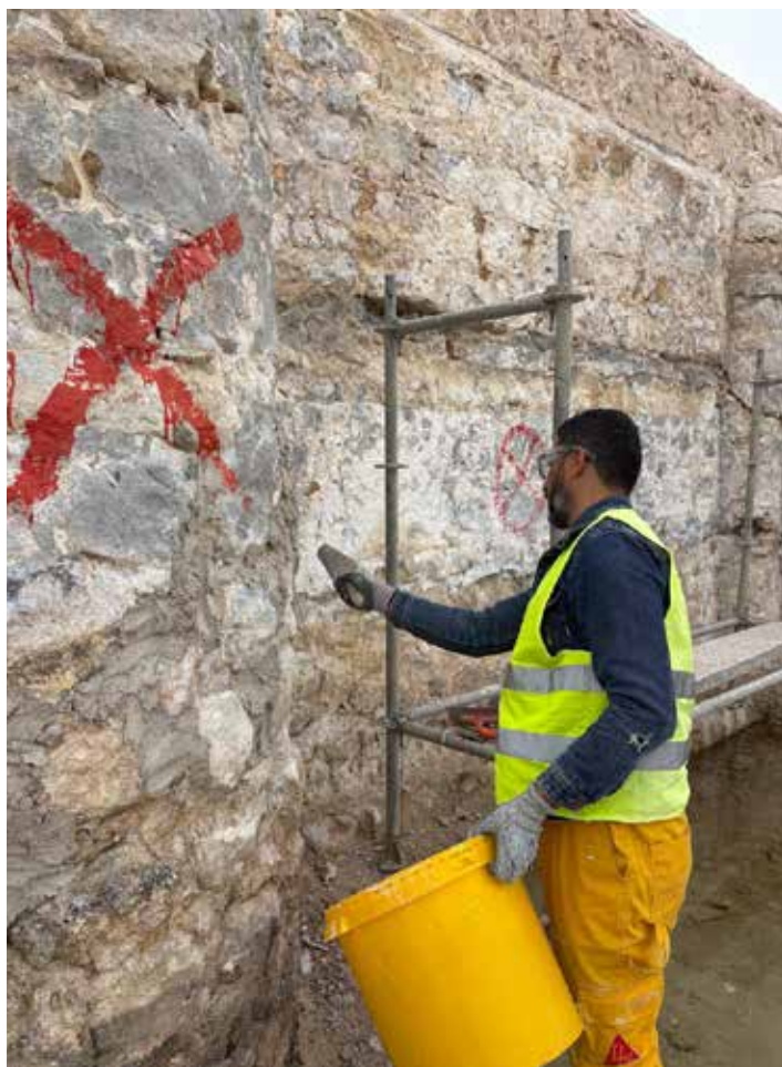
Application of the Sika CarboDur®Grid+ SikaEmaco®S 285 TIX System.
